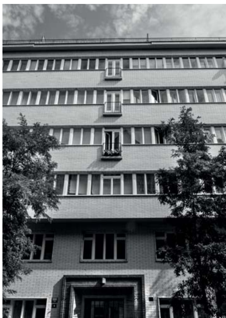
Apartment block in Baranova Street, Prague, Lagus and Wels, 1938–1939 / photo © Karel Cudlín
