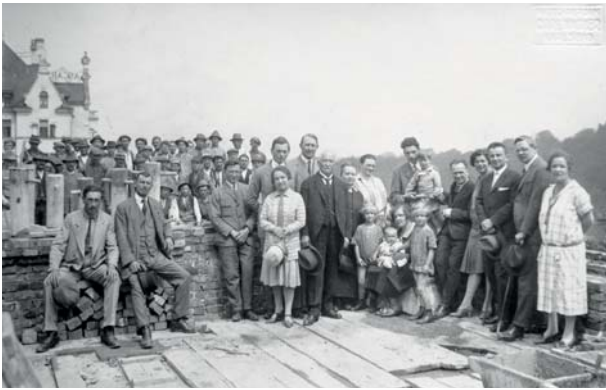
The Gea apartment block under construction, Karlovy Vary, 1928. Rudolf is standing third from right.
